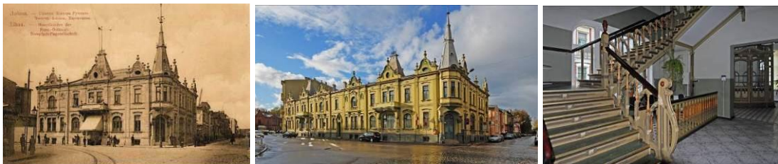
Fig. 2. Russian-Asian Steamer Shipping Company offices at Kūrmājas prospekts 2/4/6. Attributed to L. Melville. 1908–1911. Postcard of 1908, photograph of the building (J. Krastins, 2011) and vestibule (photograph by J. Krastiņš, 2012)
