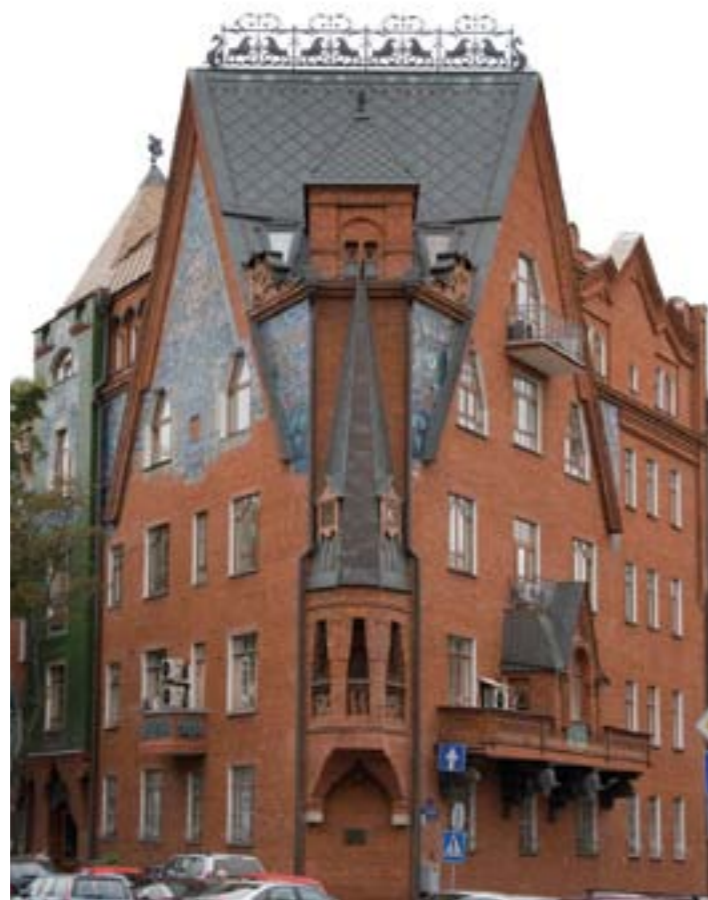
Pertsov apartment building, 1906-1910, by engineer N.K. Zhukov and designer S.V. Maliutin
