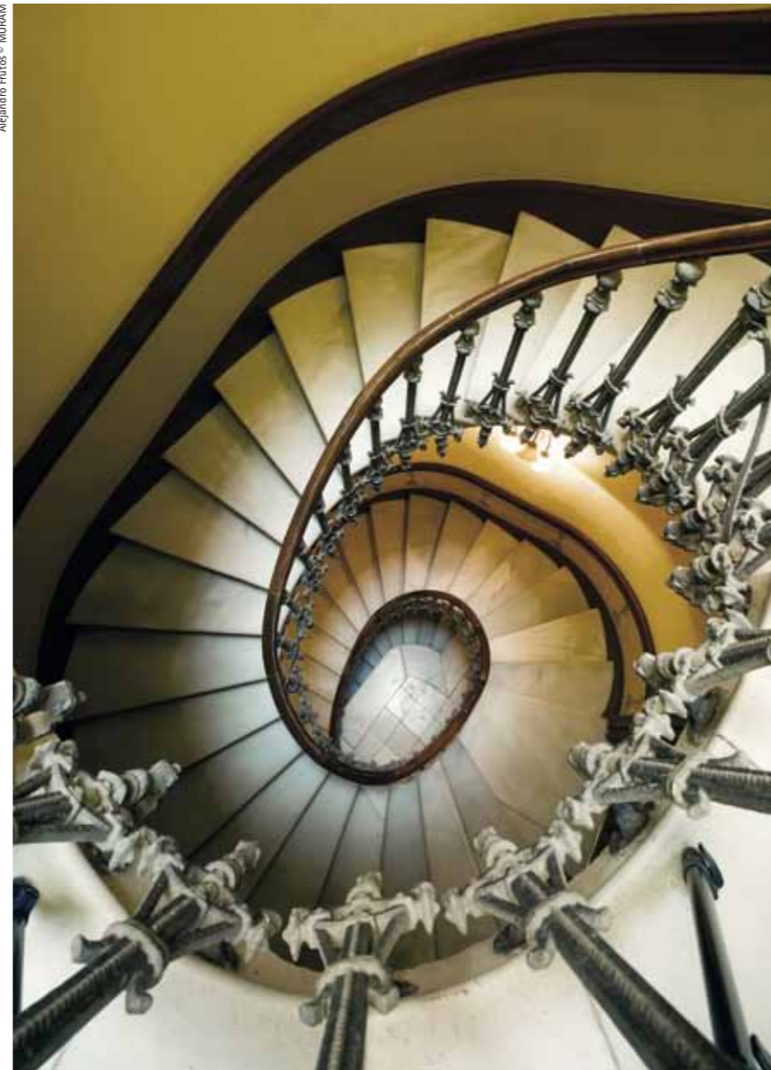
Spiral staircase seen from above Vista zenital de l'escala de cargol
