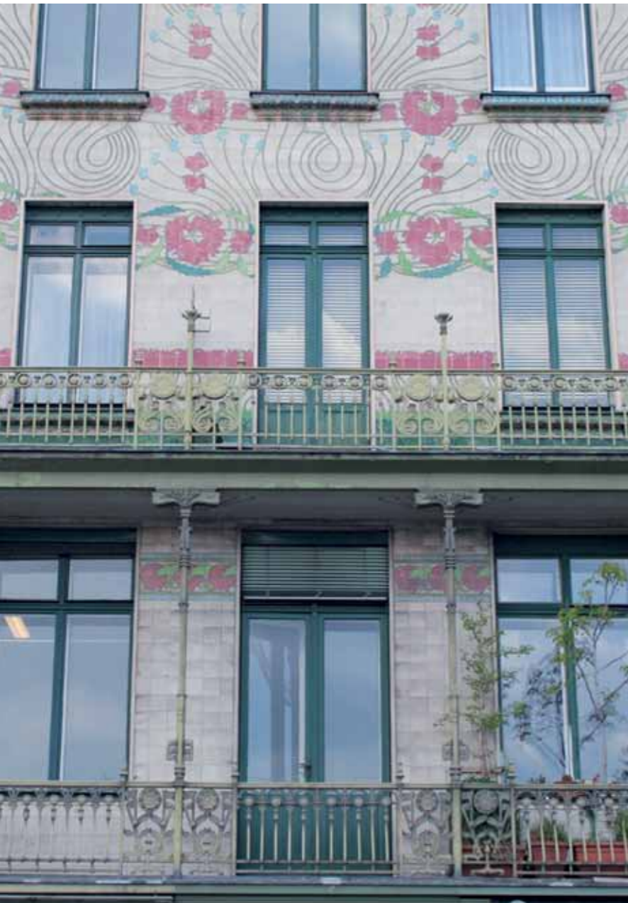
Otto Wagner, 1898-1899. Majolica tiles designed by Alois Ludwig, on the Majolikahaus's façade
