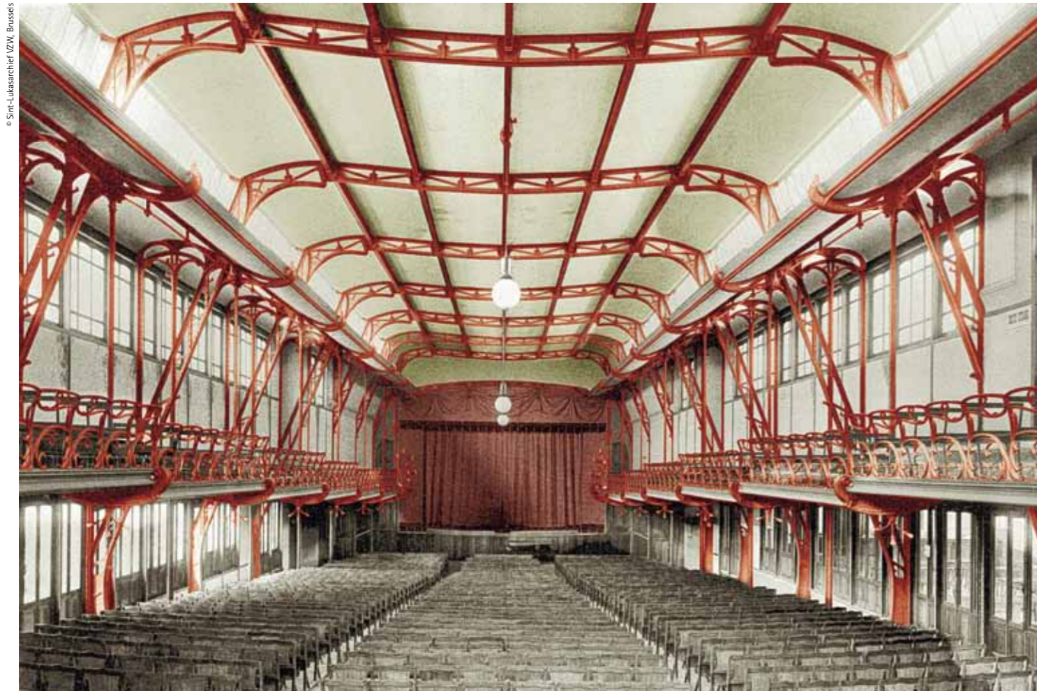
Computer simulation of the famous Maison du Peuple, showing its characteristic red iron structures
