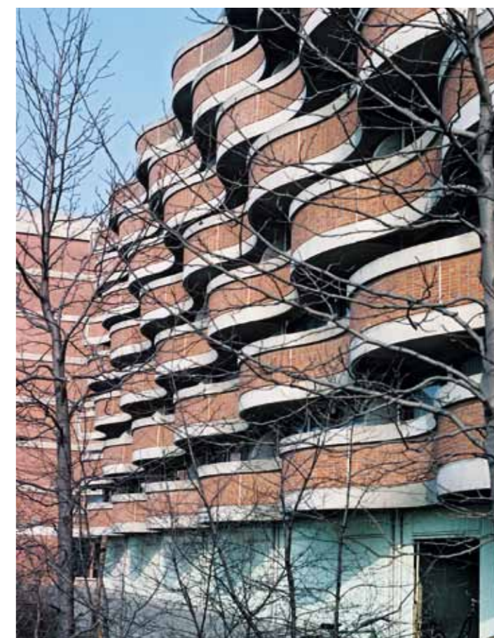
In 1969 the architect Renaat Braem wrote an essay titled: "Art Nouveau and Us", and subsequently his modernistic style evolved to more organic solutions, as in this social housing project of 1977 in the Belgian town of Boom
