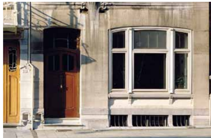
The original ground-floor window of the workshop building was recovered after a painstaking study and design process. Far top, this period picture from the Horta Museum archive was a crucial document in the process; above this caption, the altered window in 1998, before it was restituted. Below right, design by Barbara Van der Wee for the reproduction of the wrought-iron railing by Luc Reuse, and below left, the reproduced railing was finally set in place in 1991
