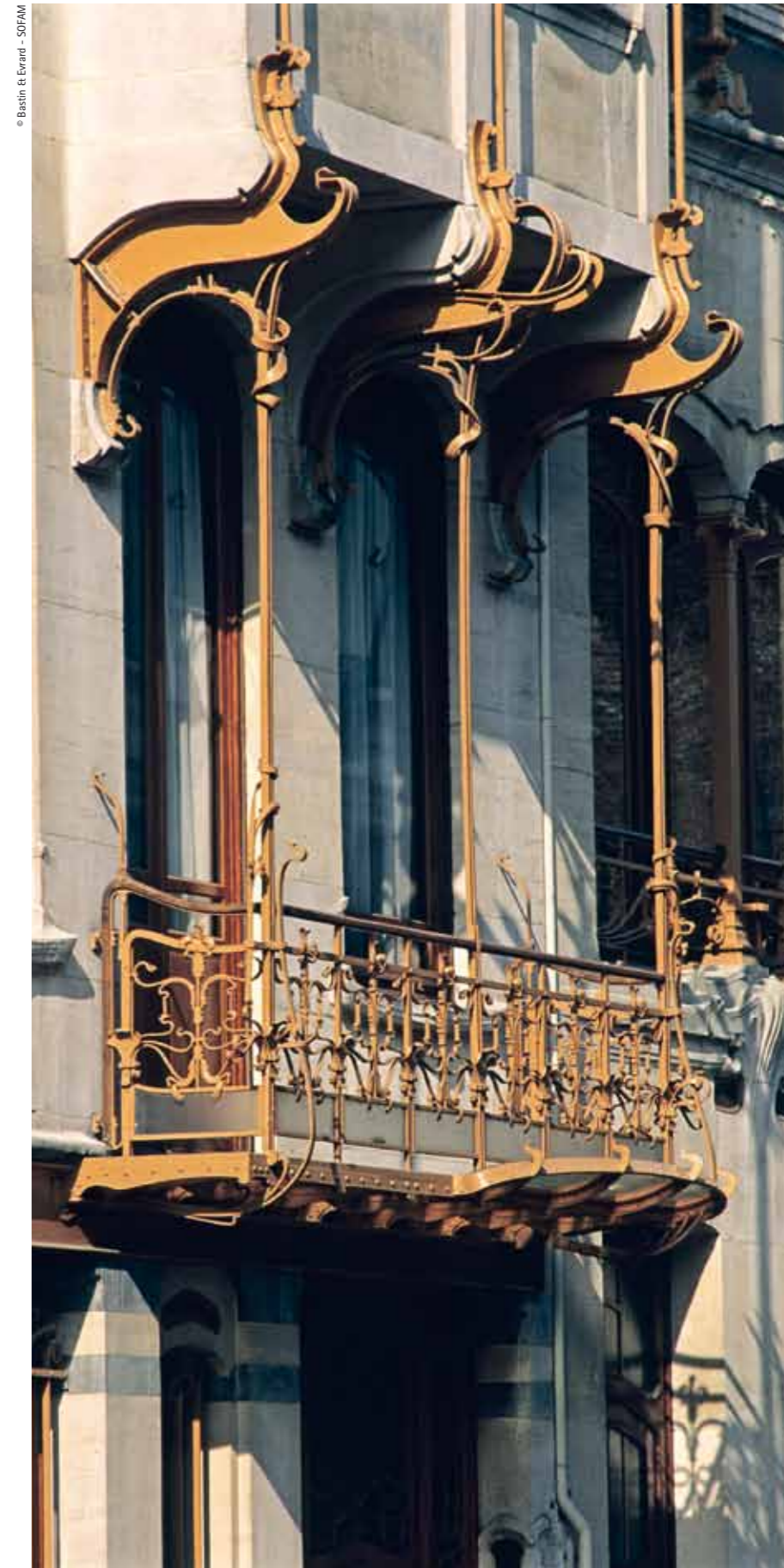
Thorough stratigraphic and archival research enabled the original colours of the woodwork and wrought-iron elements of the façade to be identified and recovered
